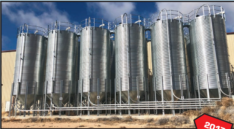
(12) CORRUGATED GALVANIZED STEEL SILOS
