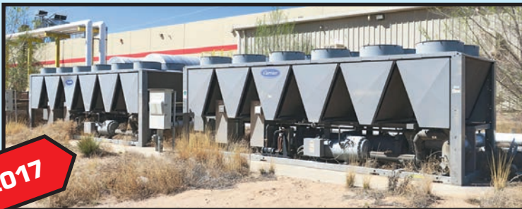
(2) CARRIER AIR-COOLED SCREW TYPE LIQUID CHILLERS
