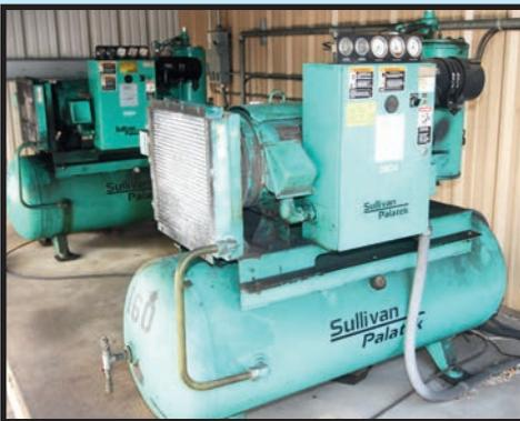
(2 OF 4) SULLIVAN PALATEK MDL. 25D4 ROTARY SCREW AIR COMPRESSORS
